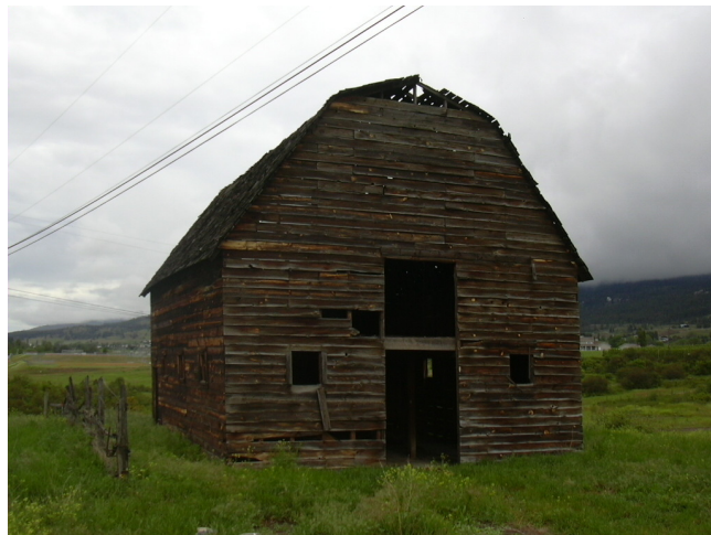
Figure 1. Buildings at 4310 Old Vernon Road, Kelowna, BC
